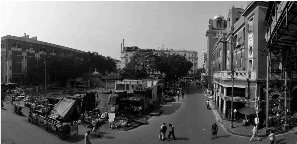
Figure 2. Chaplin cinema demolished during May 2013.
