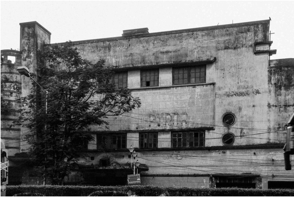
Figure 15. Purna cinema façade.
